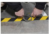
If you are laying PM Anti-Slip 3406 conformable, please use a rubber mallet to fit it to the structure of the surface.
