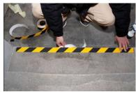
length, remove liner partly, angle the tape (keep a distance of 15 mm from the leading edge of stairs to avoid damage of the tapes' edges), take-off the remaining liner and press on the tape.
