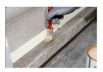
**4.** Brush blowy, sucking surface with Anti-Slip Primer (in any case when using it outdoor!).
